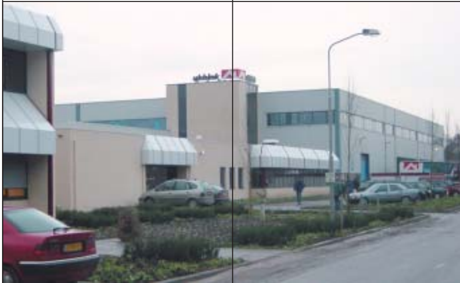
Modern and welcoming – Ubbink's headquarters in Doesburg, NL
