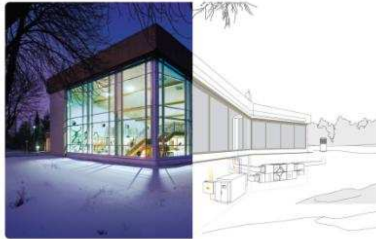
CHP and Air conditioning with heat recovery
